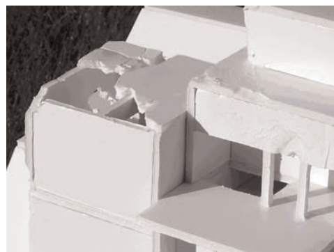
collapsed roof (detail)
